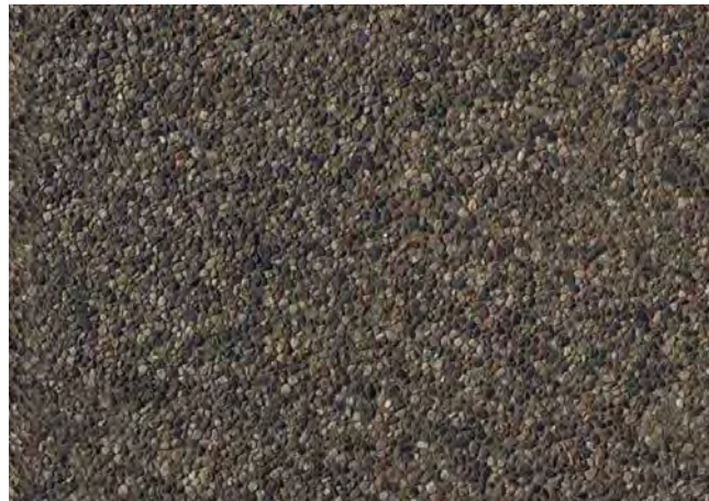
Exposed coarse aggregate finish.
