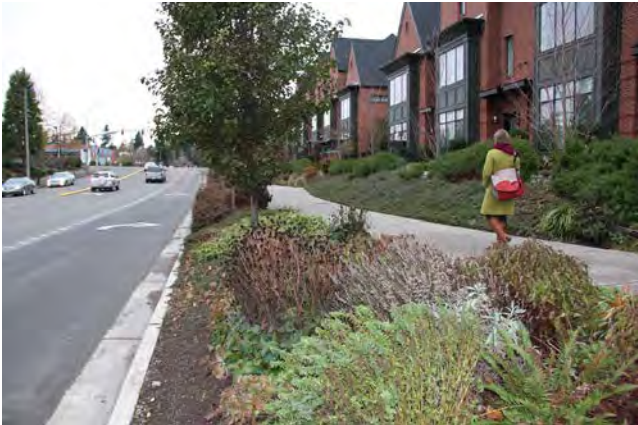
Ribbon sidewalk on NE 12th Street, Bellevue, WA
