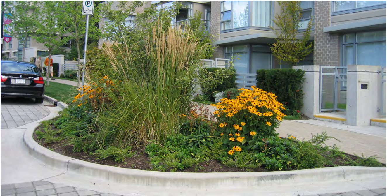
Curb extensions with plantings at UniverCity, BC. Courtesy of Carl Sundstrom, PBIC
