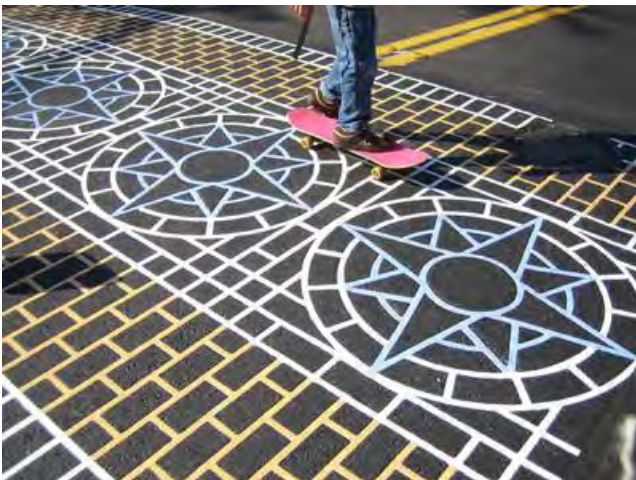
Asphalt sidewalk with thermoplastic imprinted pattern. Courtesy of www.streetprint.com
