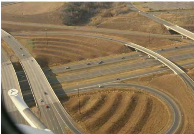
Earthwork as monumental gateway. © 1980 Andrew Leicester, Cloverleaf
