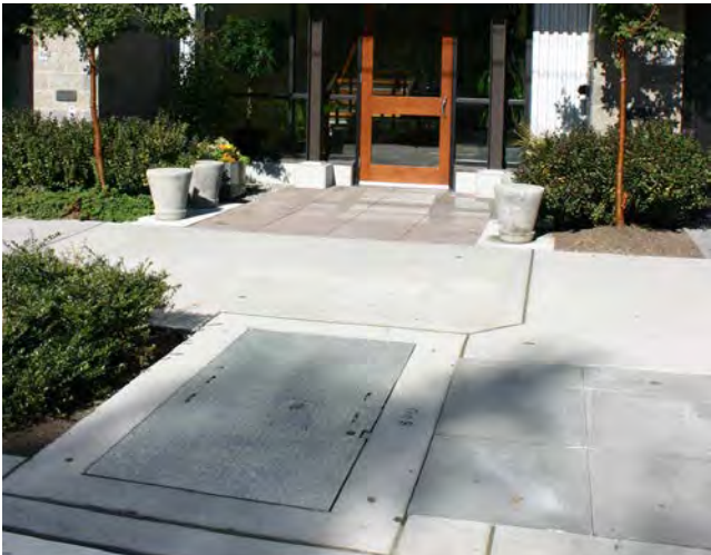
Subgrade utility vaults located outside of clear walk space and planter walkway. Seattle, WA.
