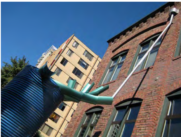
Captured rainwater held in cistern and redirected to plants. © 2003 Buster Simpson, Beckoning Cistern
