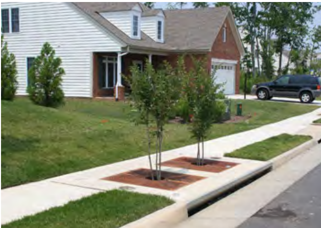
Stormwater treatment within an urban right of way. Courtesy of www.filterra.com
