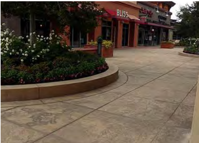
Decorative concrete at the Dos Lagos outdoor mall, CA. Courtesy of concretenetwork.com
