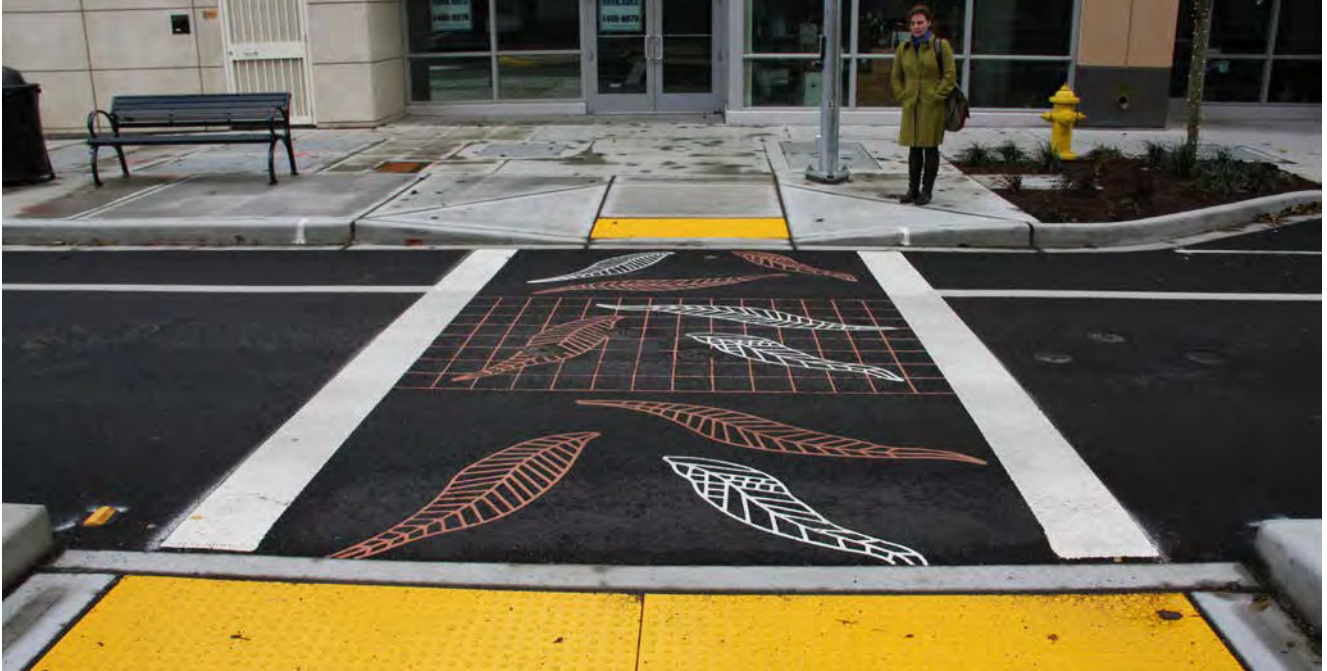
Detail of asphalt sidewalk with imprinted pattern in Downtown Bellevue
